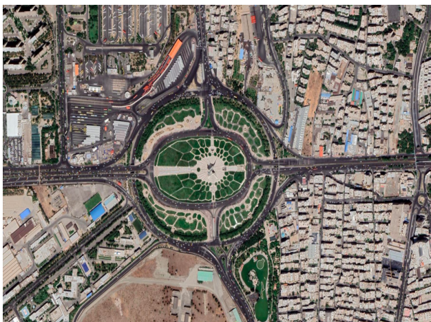
Figure 4. Aerial view of Azadi Square.
